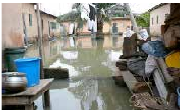
Photo 1: Flooded house in Lome/Be District
