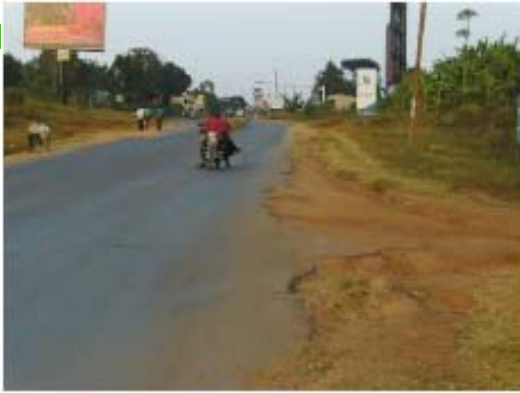
Road where uncontrolled stormwater flows in high rainfall events
