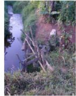
Attempts at stormwater control
