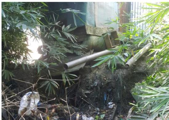
Figure 4.21: Improper discharging of liquid waste
