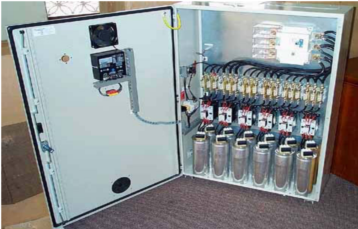
Figure 4 An automatic capacitor bank in a metal case
